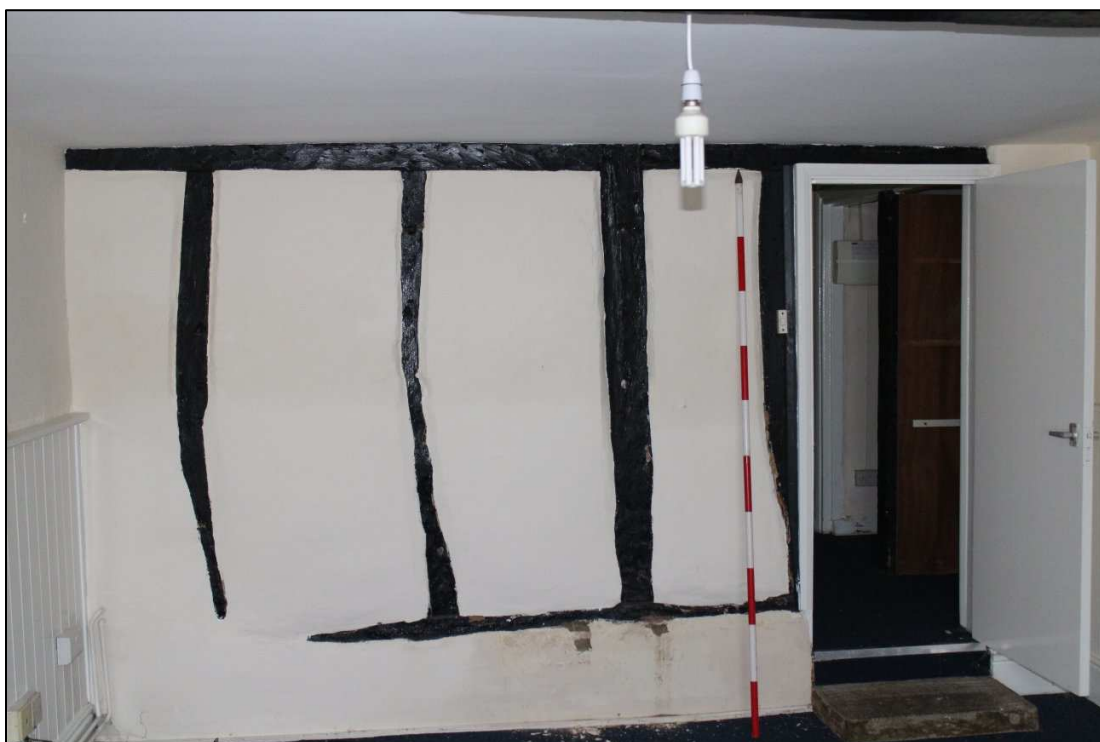
Image 11: Interior, Room G2
