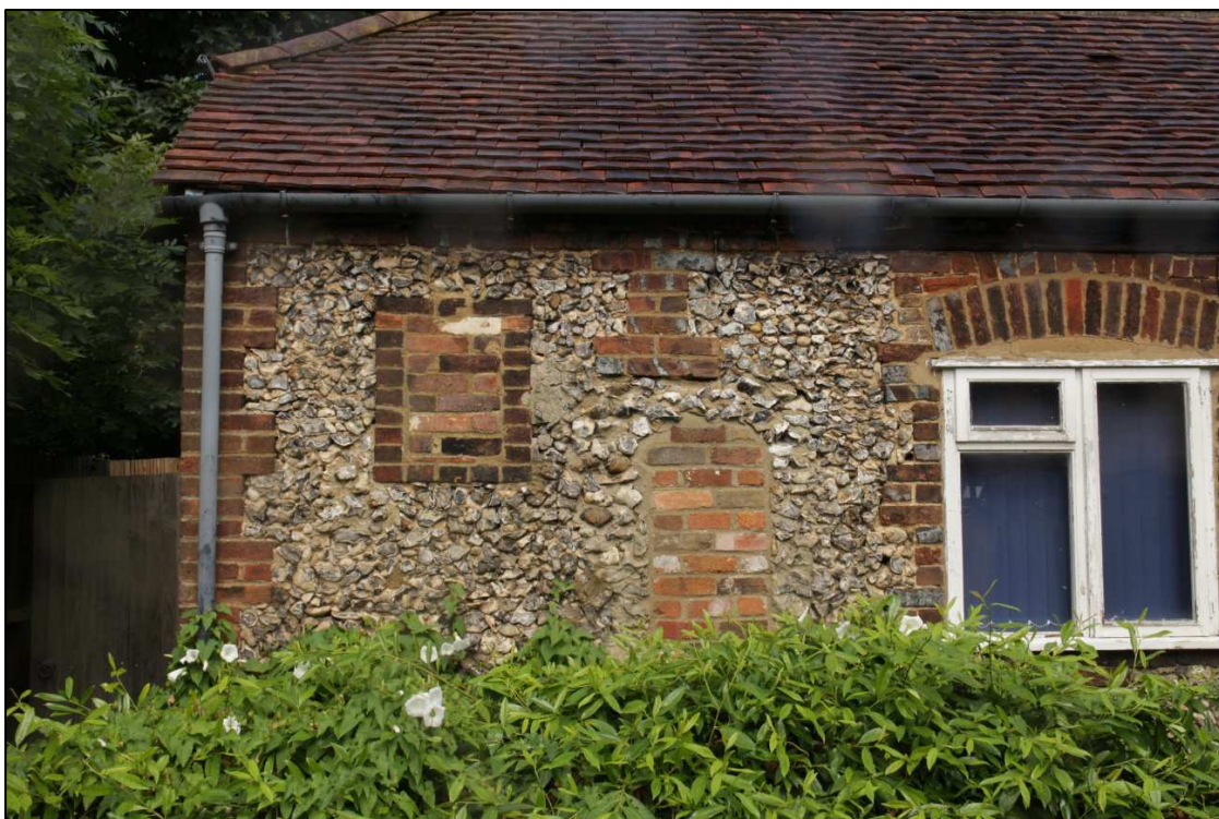
Image 7: Exterior, south-east elevation of south range
