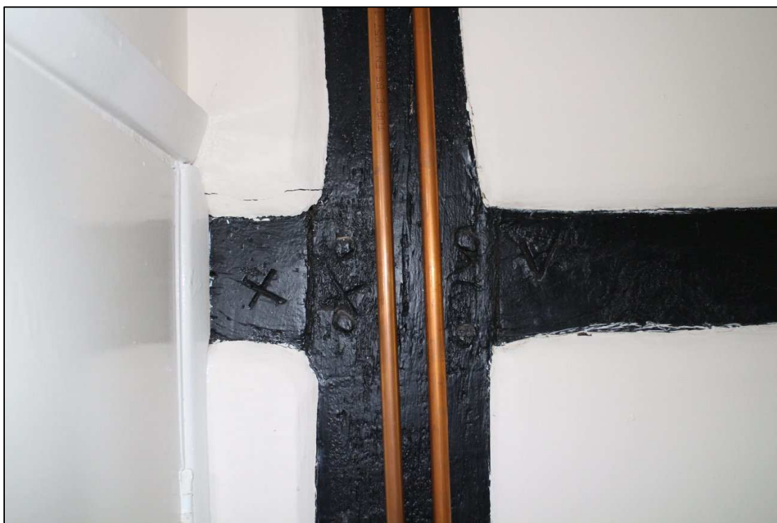
Image 16: Interior, Room G7
