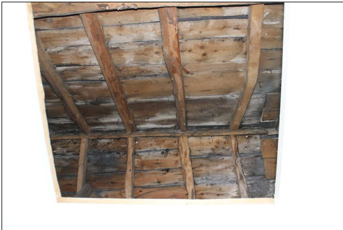
Image 14: Interior, Room G4 roof space
