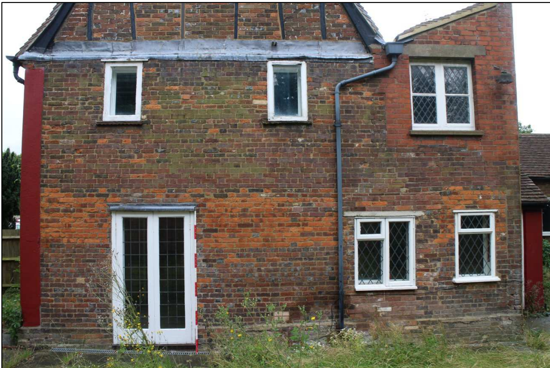
Image 3: Exterior, north-west elevation
