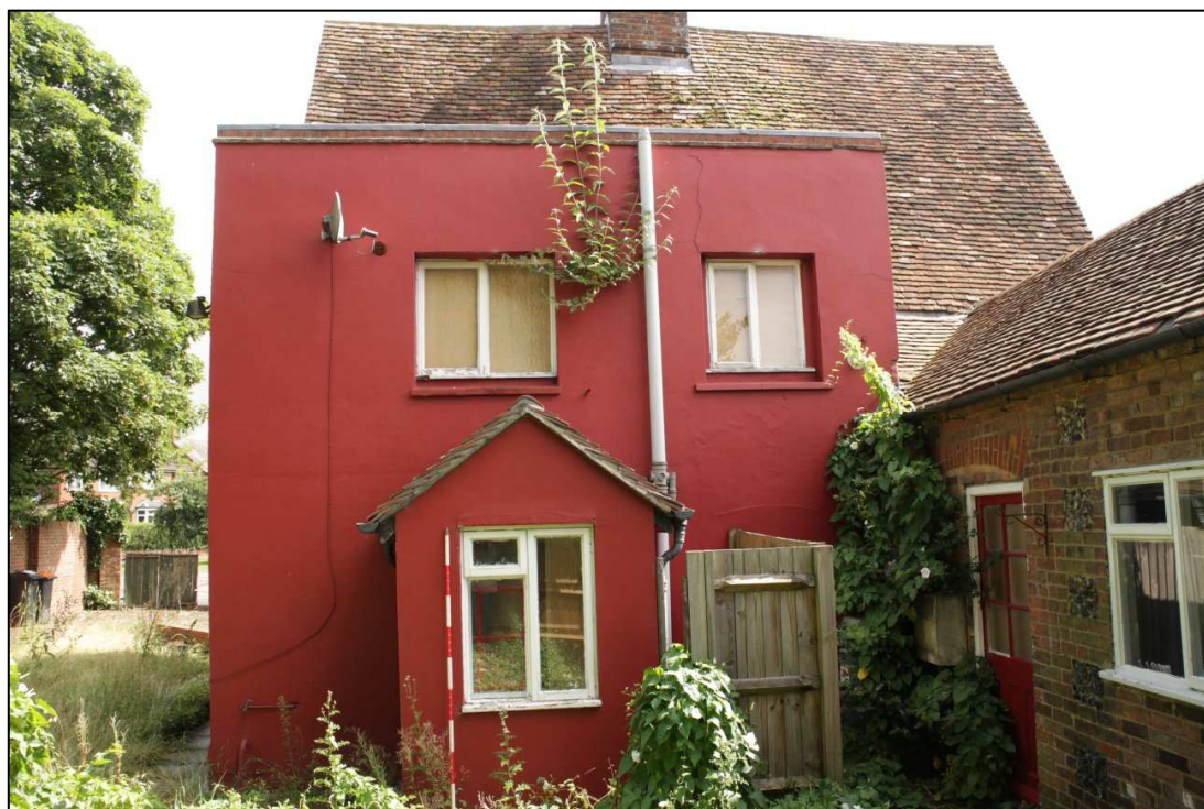
Image 5: Exterior, rear elevation
