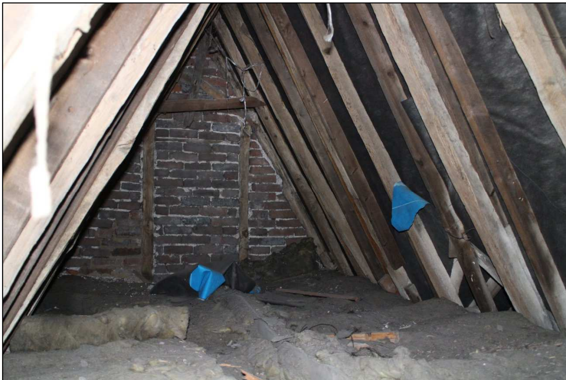
Image 25: Interior, roof space over primary range
