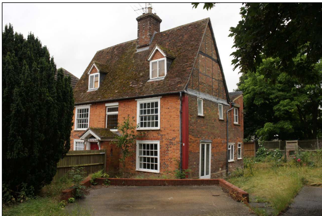
Image 1: Exterior, front elevation Showing front and north-west elevations
