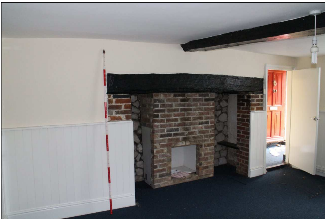
Image 10: Interior, Room G2
