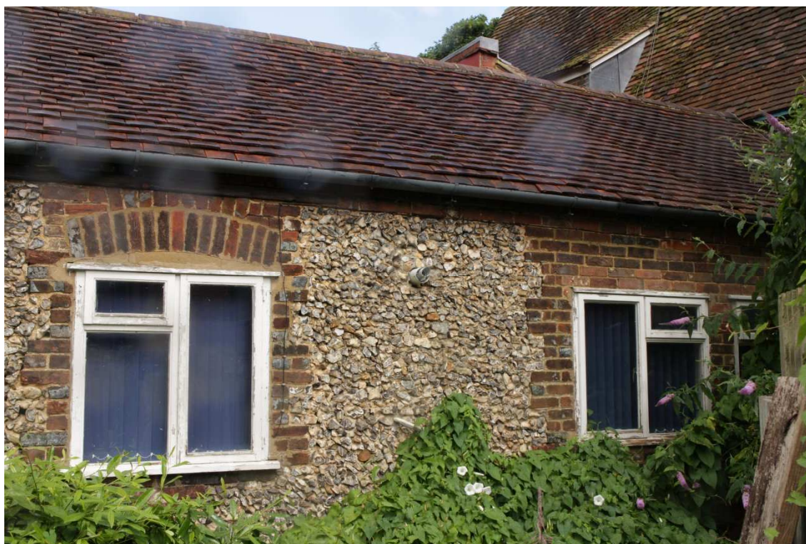
Image 8: Exterior, south-east elevation of south range
